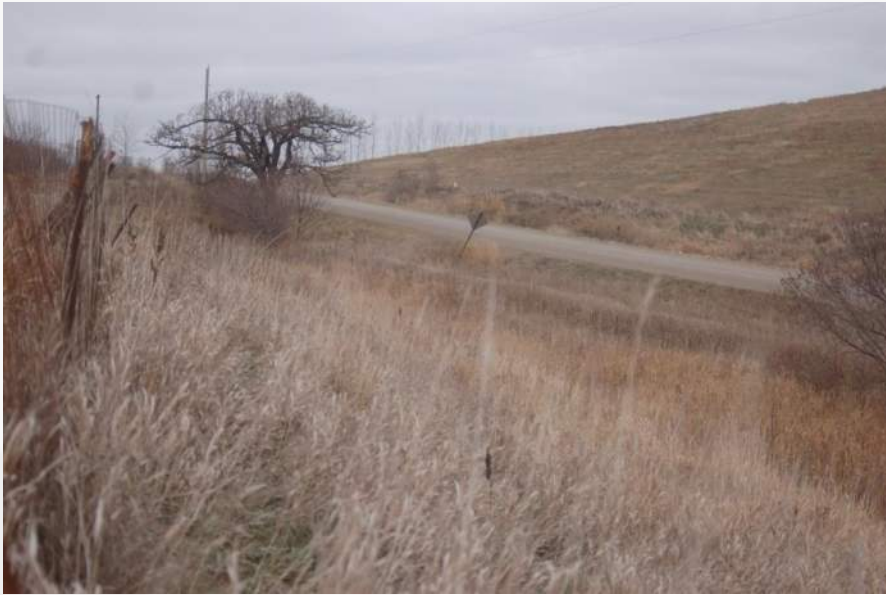
Photo 33 - Phase 2 East Exterior Slope
