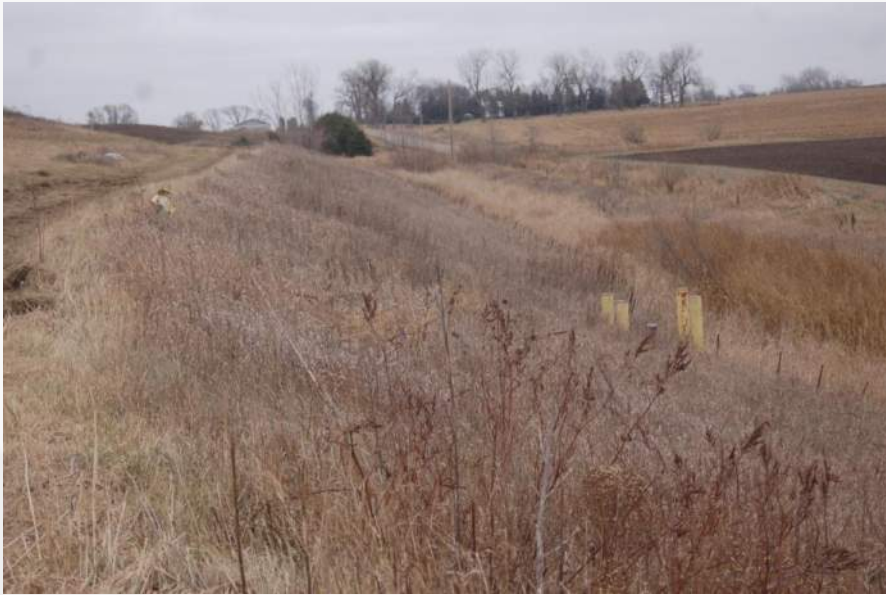
Photo 17 - Phase 2 South Exterior Slope
