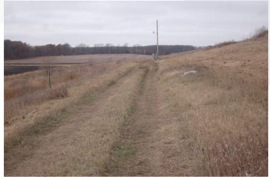
Photo 20 - Phase 2 Top South Berm
