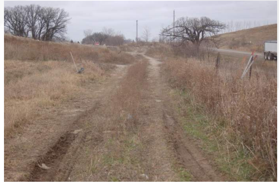
Photo 34 - Phase 2 Top East Berm
