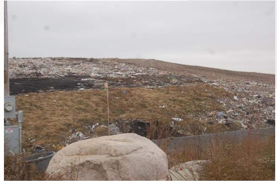
Photo 2 - Phase 3 North Temp Berm
