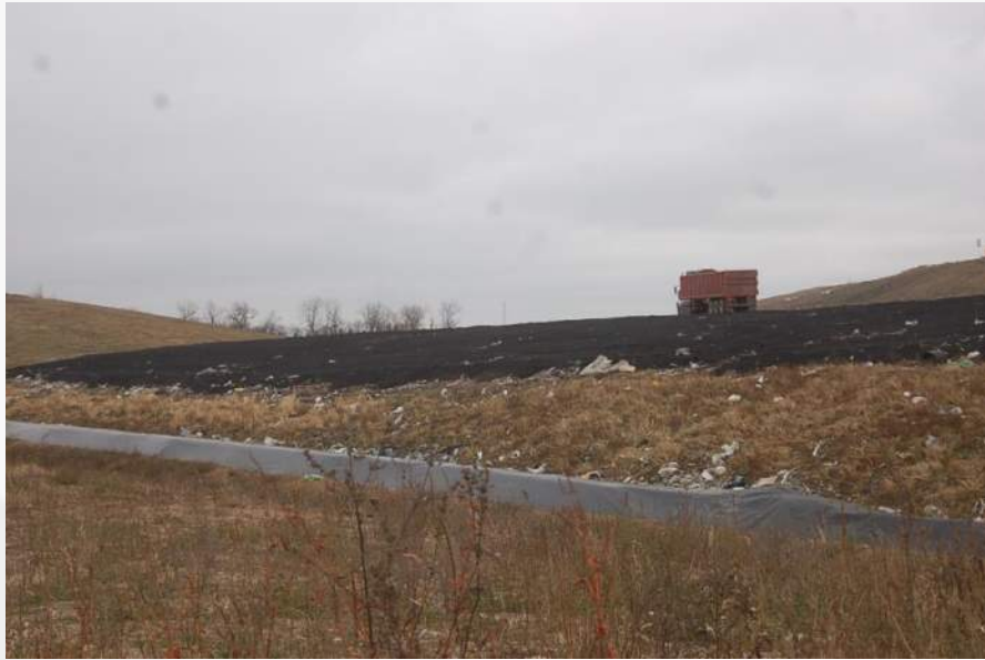
Photo 1 - Phase 3 North Temp Berm
