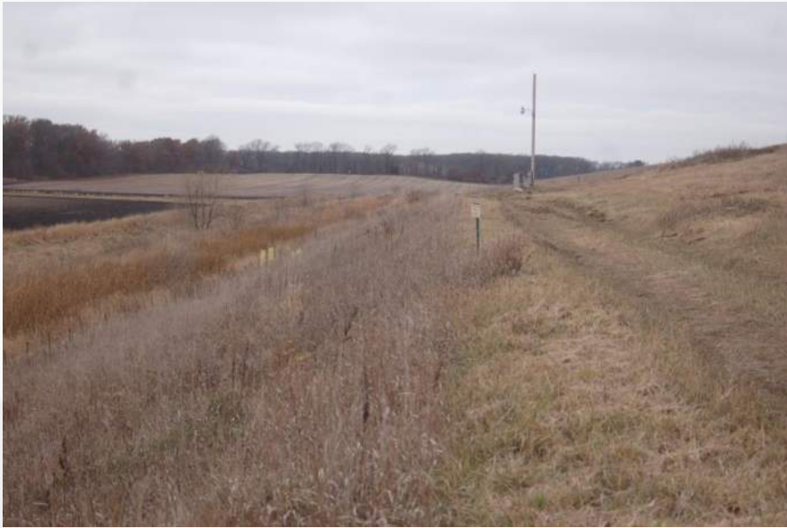
Photo 21 - Phase 2 South Exterior Slope
