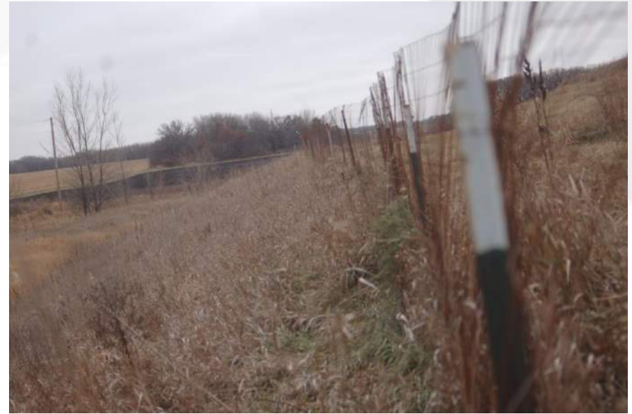
Photo 32 - Phase 2 East Exterior Slope
