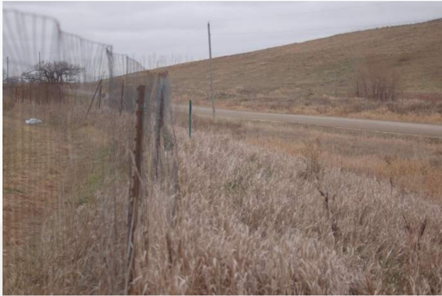
Photo 29 - Phase 2 Top East Berm
