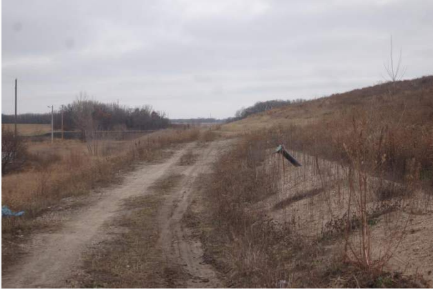
Photo 37 - Phase 2 Top East Berm
