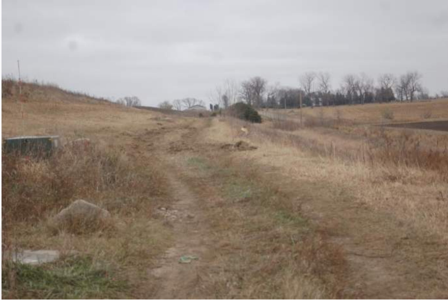
Photo 15 - Phase 2 Top South Berm
