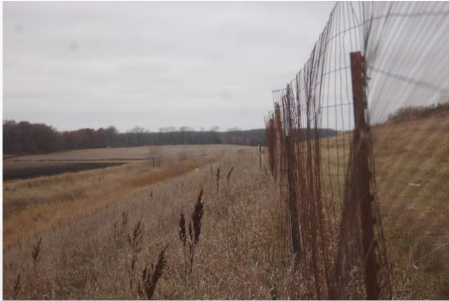
Photo 27 - Phase 2 South Exterior Slope
