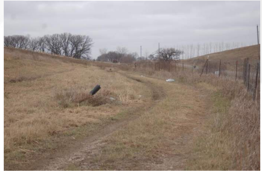
Photo 28 - Phase 2 East Exterior Slope
