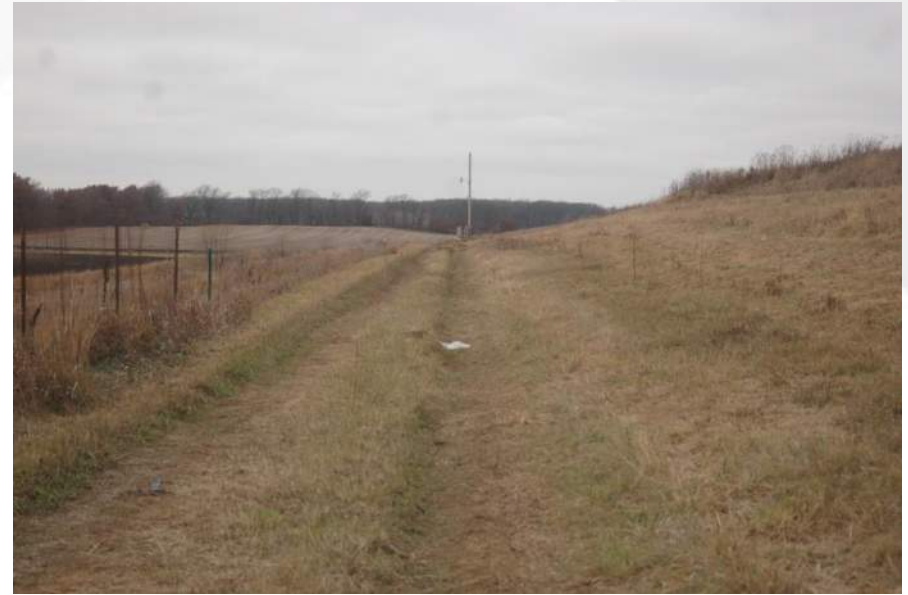
Photo 26 - Phase 2 Top South Berm
